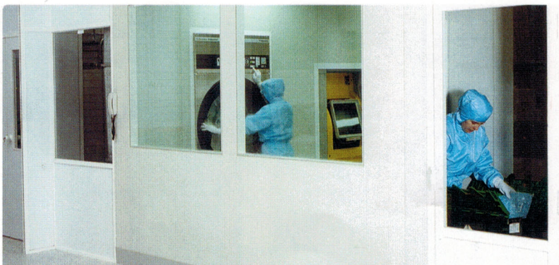
Partial exterior view - SAS clean material output.
